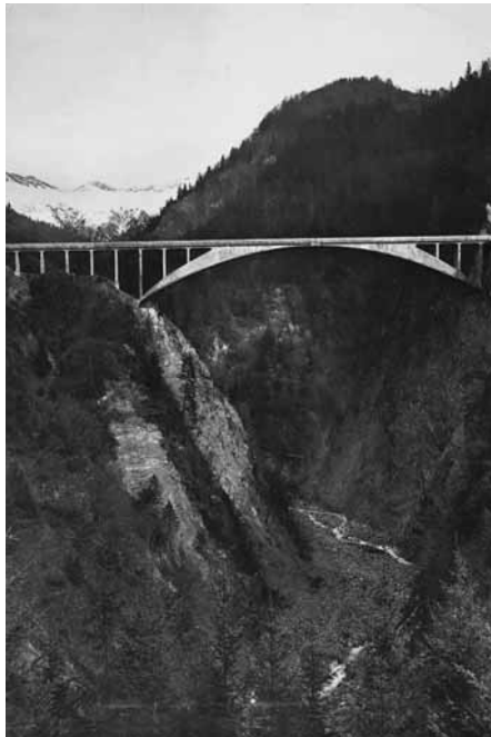
Salginatobel Bridge, Switzerland, built 1929–30.
