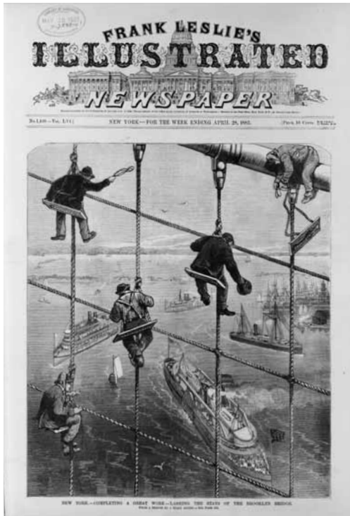
Workers on the cables of Brooklyn Bridge, 1883.
