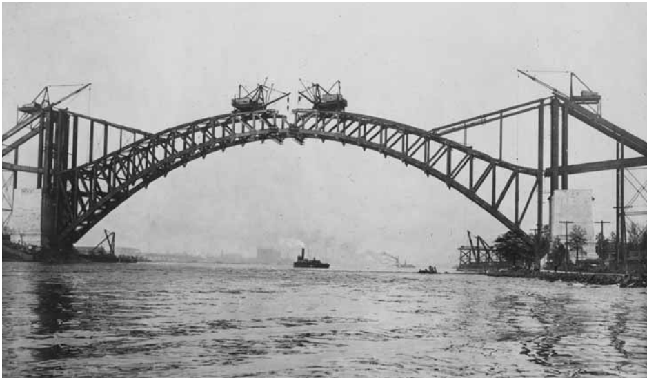
Hell Gate Bridge, New York, under construction, 1915.
